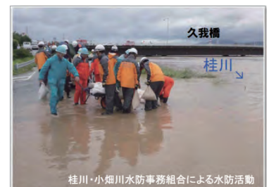
Even attenuated flood water overtopped embankment. Flood fighters are building up sand bags (photo from Kinki R.B., MLIT)
