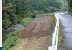
Sediment Replenishment, Nunome dam
