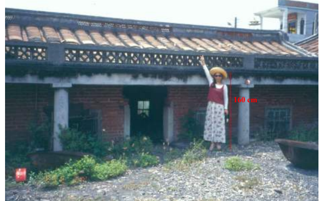
A house in an area where land subsidence is severe due to overpumping of groundwater
